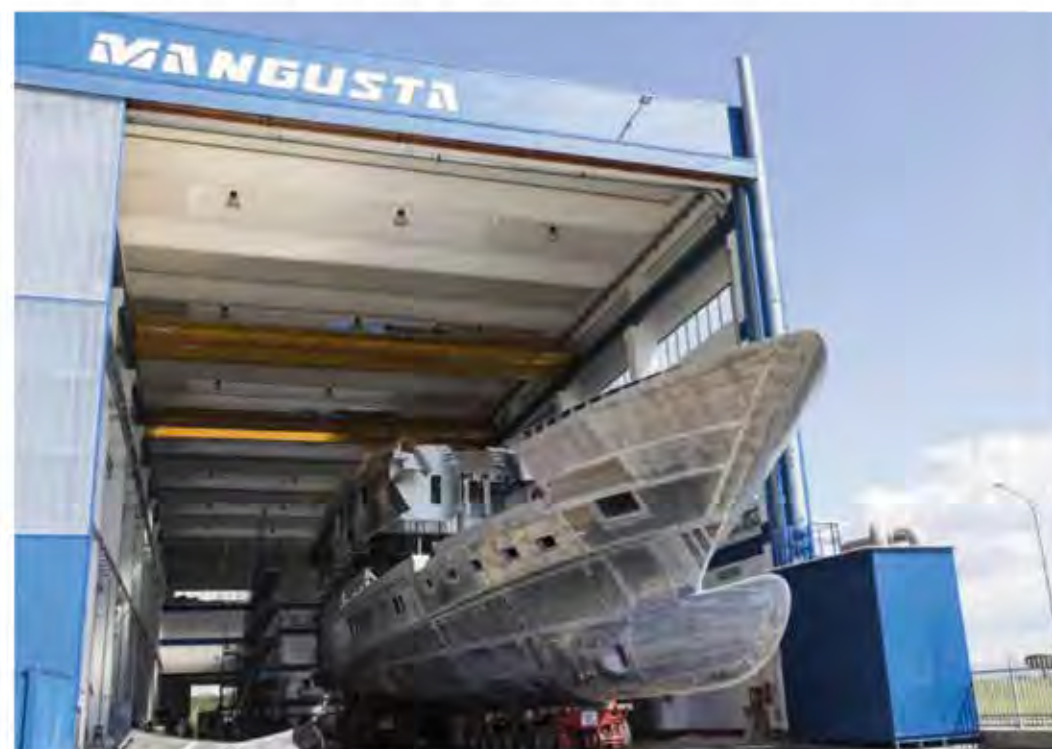
Mangusta Gransport 45 under construction
